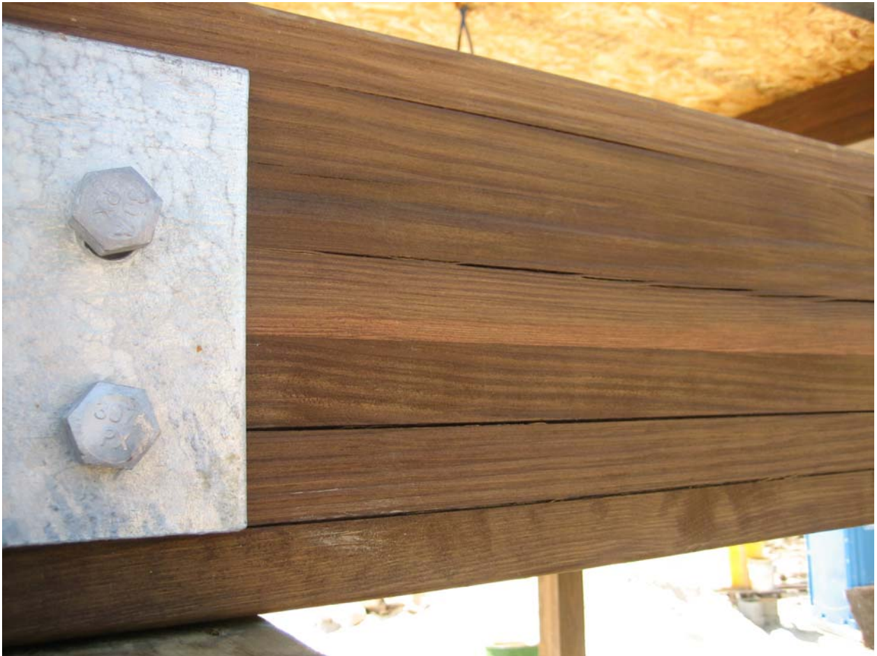
Figure 1. Checking on glulam beam treated with ACQ after bonding.
